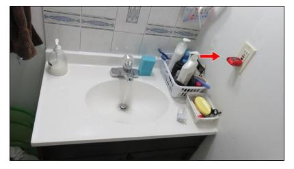
**6.4** Basement washroom GFCI not in working condition when tested, unsafe, needs to be replaced at the earliest possible.
