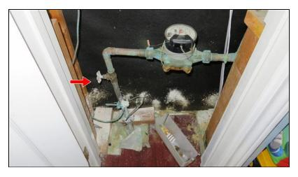
7.3 Main water shut-off is located near electrical panel in basement.
