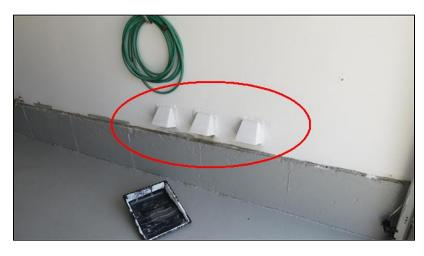
**3.2** The fire protection wall in garage is compromised by leaving basement exhaust vents in garage. This is considered unsafe until corrected. A qualified person should correct for safety.
