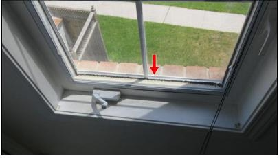
**4.5** Upstairs Jack & Jill bathroom window with sign of condensation and damaging thermal seal. The glazing between glass panes are failing at this window, needs to be replaced.
