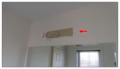
**6.3** Upstairs Jack & Jill bath vanity lights missing (left with loose wiring connections), unsafe, needs to be installed.
