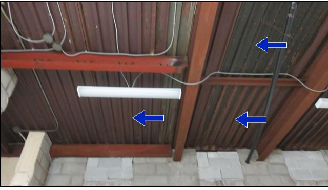
Rust Due to Leakage
