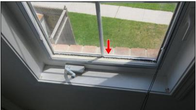
**4.5** Upstairs Jack & Jill bathroom window with sign of condensation and damaging thermal seal. The glazing between glass panes are failing at this window, needs to be replaced.
