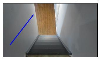
**4.3** Basement staircase handrail missing, safety hazard, needs to be installed at the earliest.
