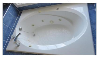
5.6 Jacuzzi tub was not in working condition, when tested. Recommended to be fixed.
