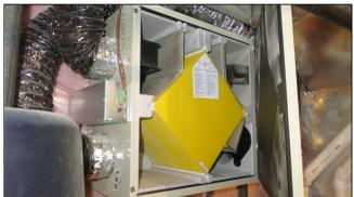
**7.4** HRV system was functional. It introduces fresh air to the building and improves climate control. Heat recovery ventilation (HRV), also known as mechanical ventilation heat recovery (MVHR), is an energy recovery ventilation system using equipment known as a heat recovery ventilator, heat exchanger, air exchanger, or air-to-air heat exchanger which employs a cross flow or counter-flow heat exchanger.
