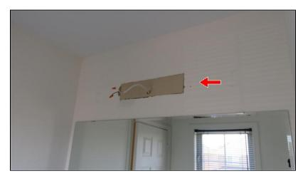
**6.4** Upstairs Jack & Jill bath vanity lights missing (left with loose wiring connections), unsafe, needs to be installed.
