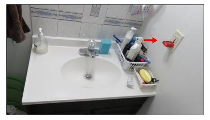
**6.6** Basement washroom GFCI not in working condition when tested, unsafe, needs to be replaced at the earliest possible.
