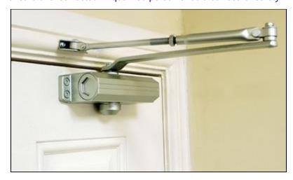
**3.5** Garage door (to dwelling unit) hydraulic door closer missing, needs to be installed. Self closing is a requirement for proper gas separation (carbon monoxide from car fumes) and for fire separation.
