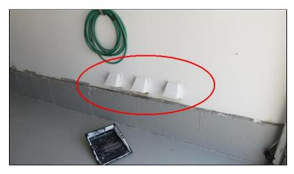
**3.4** The fire protection wall in garage is compromised by leaving basement exhaust vents in garage. This is considered unsafe until corrected. A qualified person should correct for safety.
